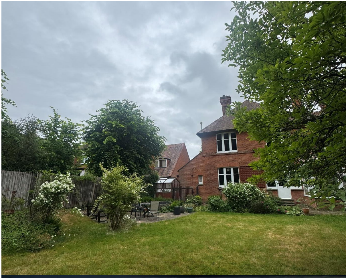
Figure 10: Rear of No. 73
