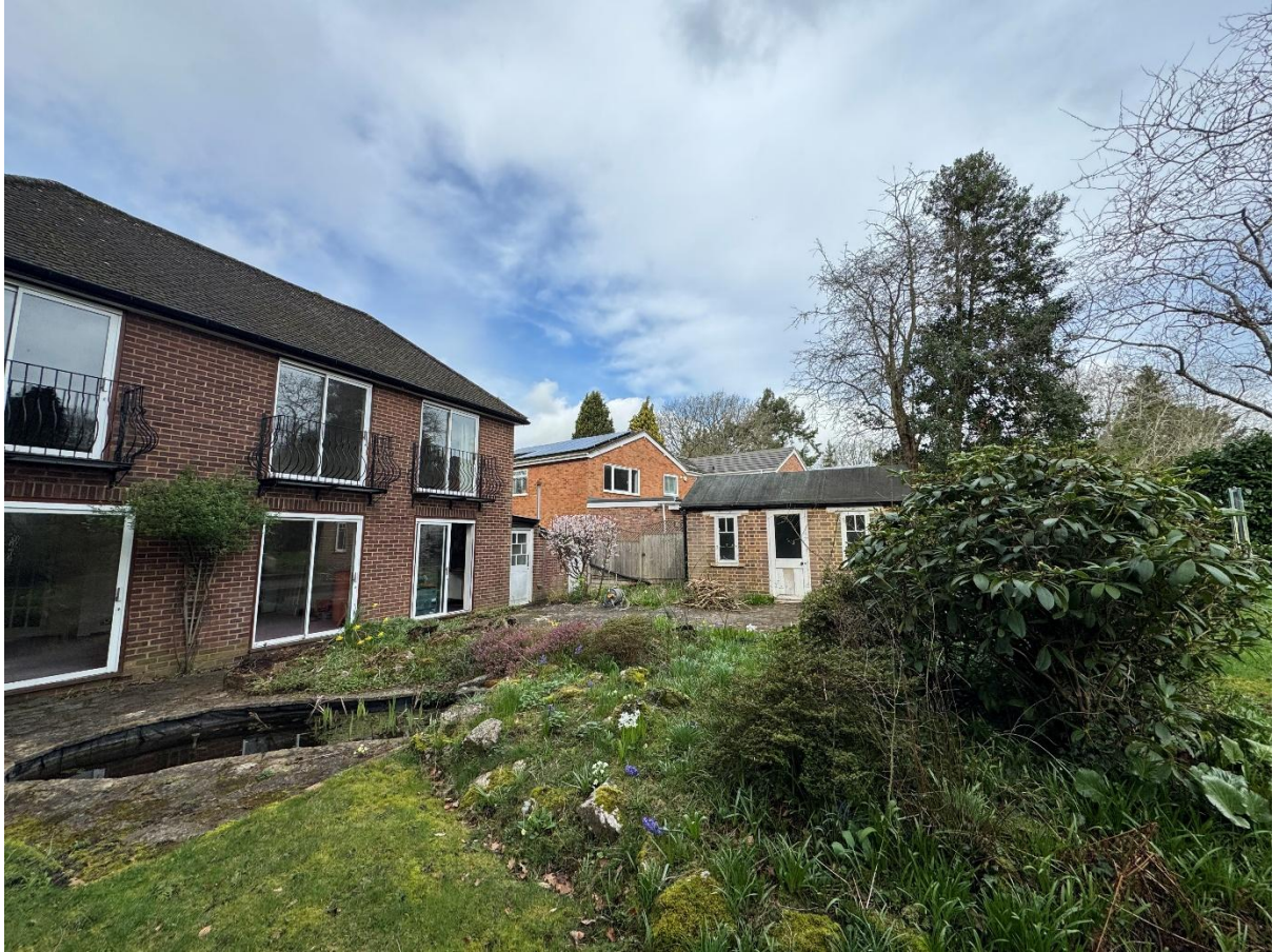
Figure 2: View of No. 18A
