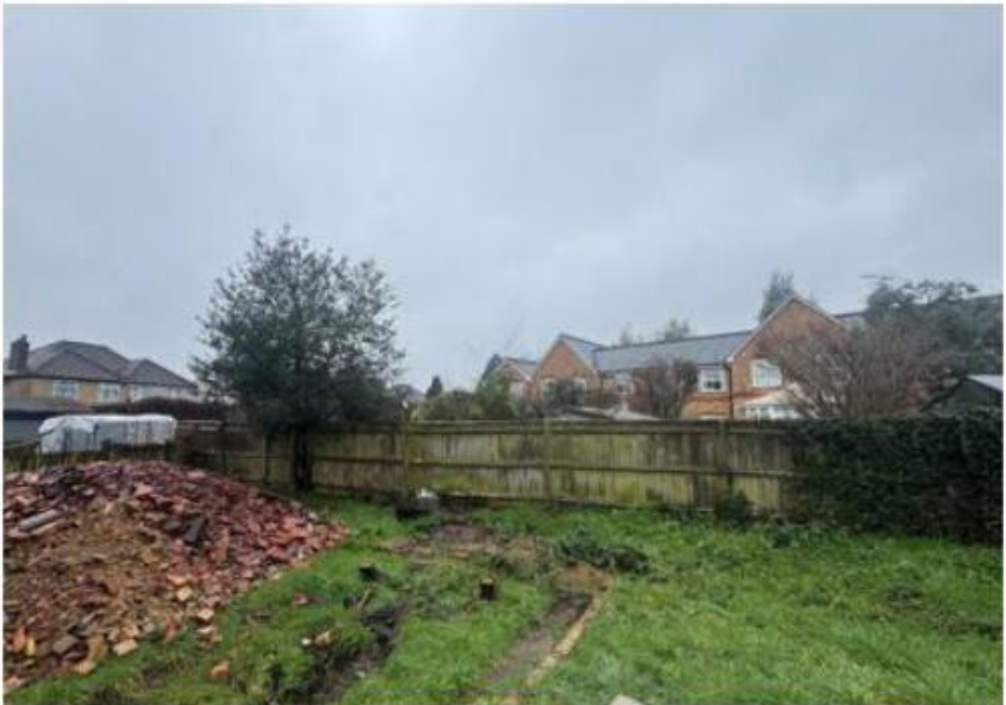
Figure 3: February 2026 Front Elevation and Rear View
