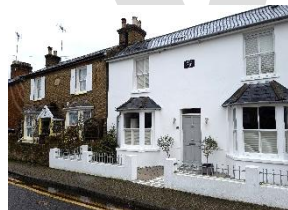
Stock brick and render with timber sash windows and panelled timber doors
