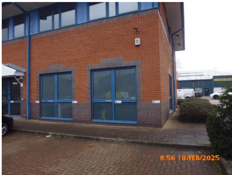
Front of Unit 8
