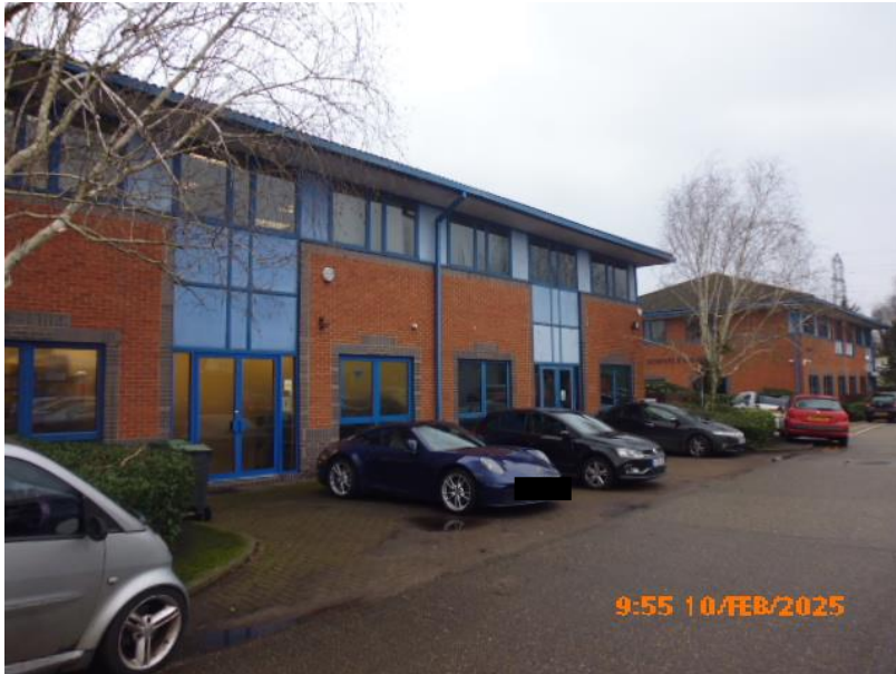
Rear of Unit 6
