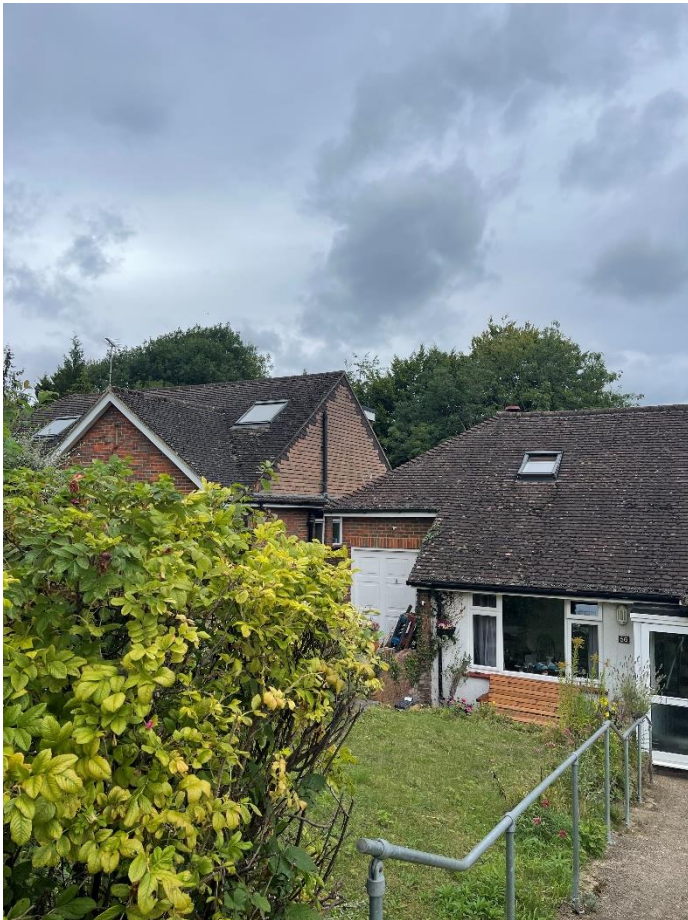
Available views of existing dormer from road (above)
