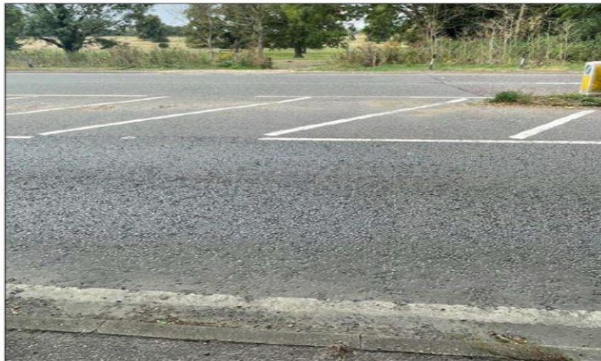
Photo 3.7 – A41 Adjacent to Future Pedestrian/Cycleway Entrance
