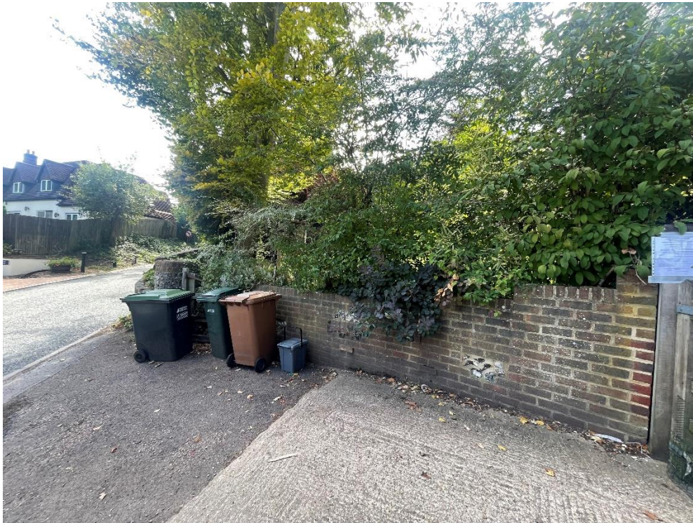
Existing retaining brick wall – indication of existing land levels.
