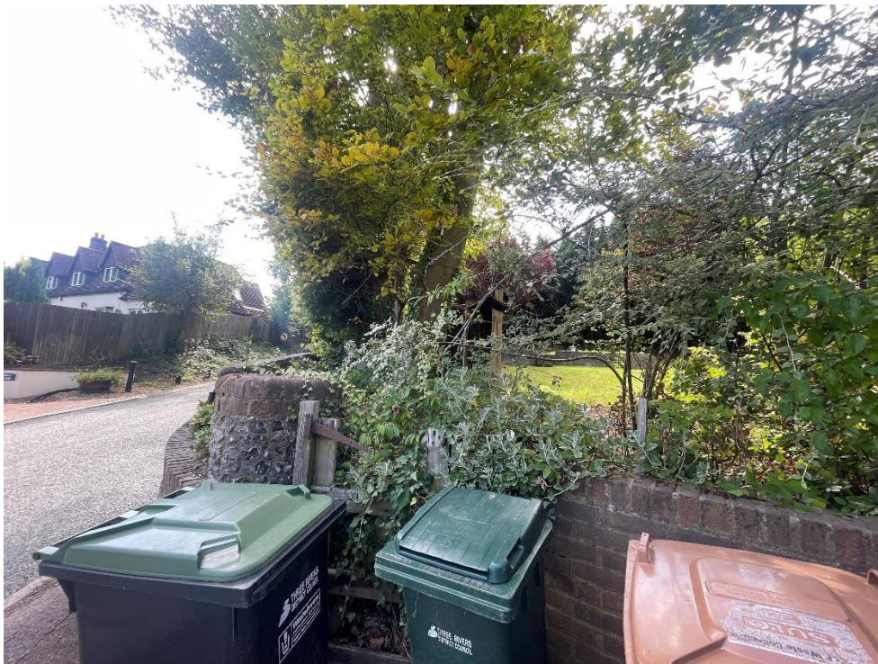
Existing retaining brick wall – indication of existing land levels. Original Brick and Flint wall to be retained.
