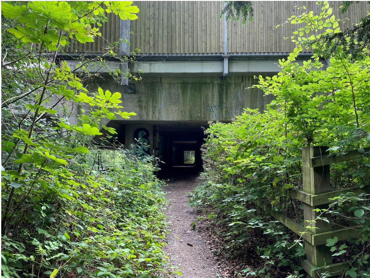
Figure 21 Underpass below the M25 in the north-east of Compartment 2
