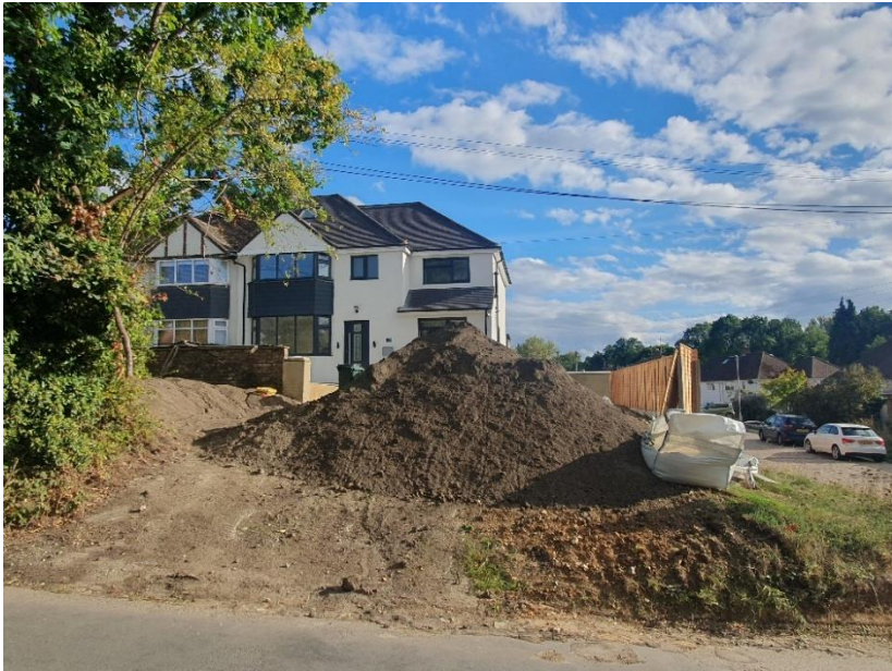
Site following commencement of works
