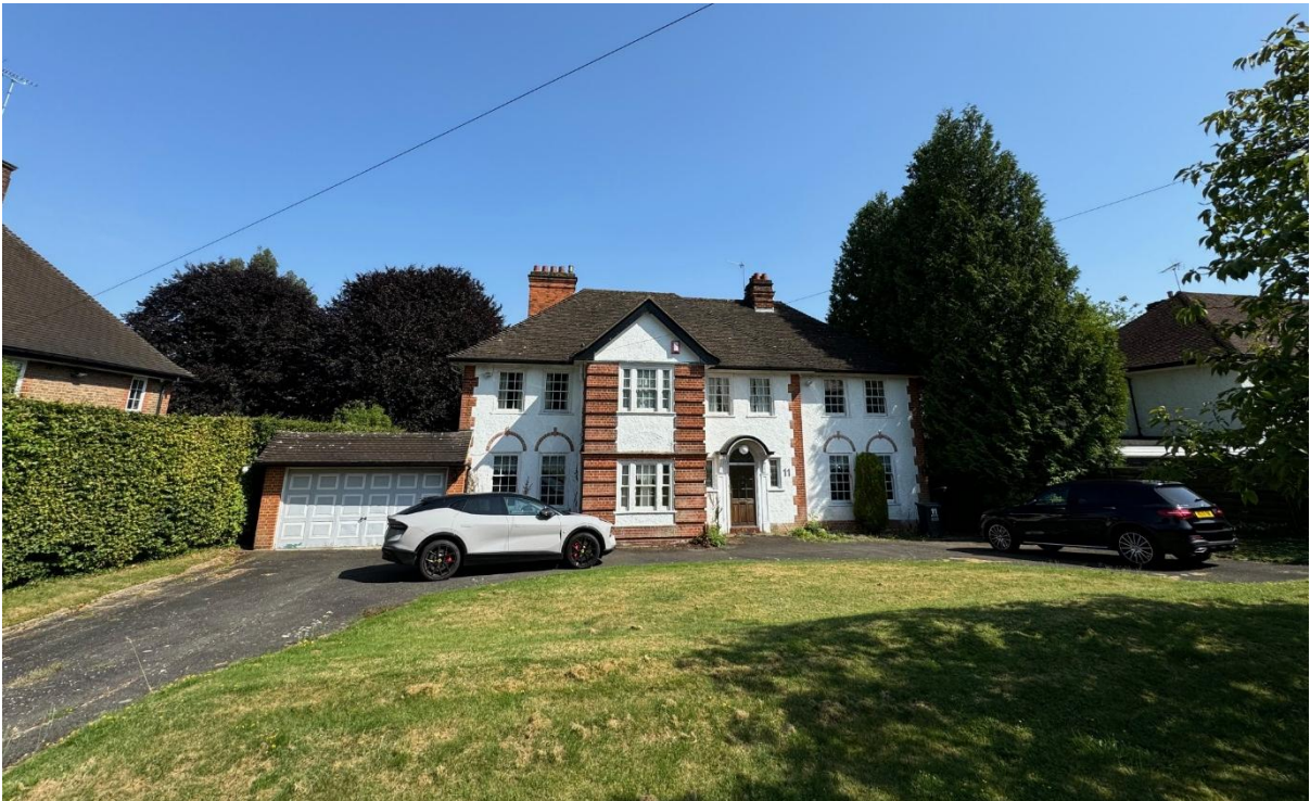
Figure 2: July 2024 Pre-existing Front Elevation
