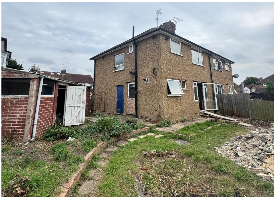
Figure 1: October 2025 Pre Existing Rear Elevation
