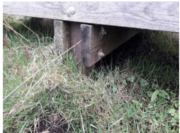
Existing boardwalk construction detail
