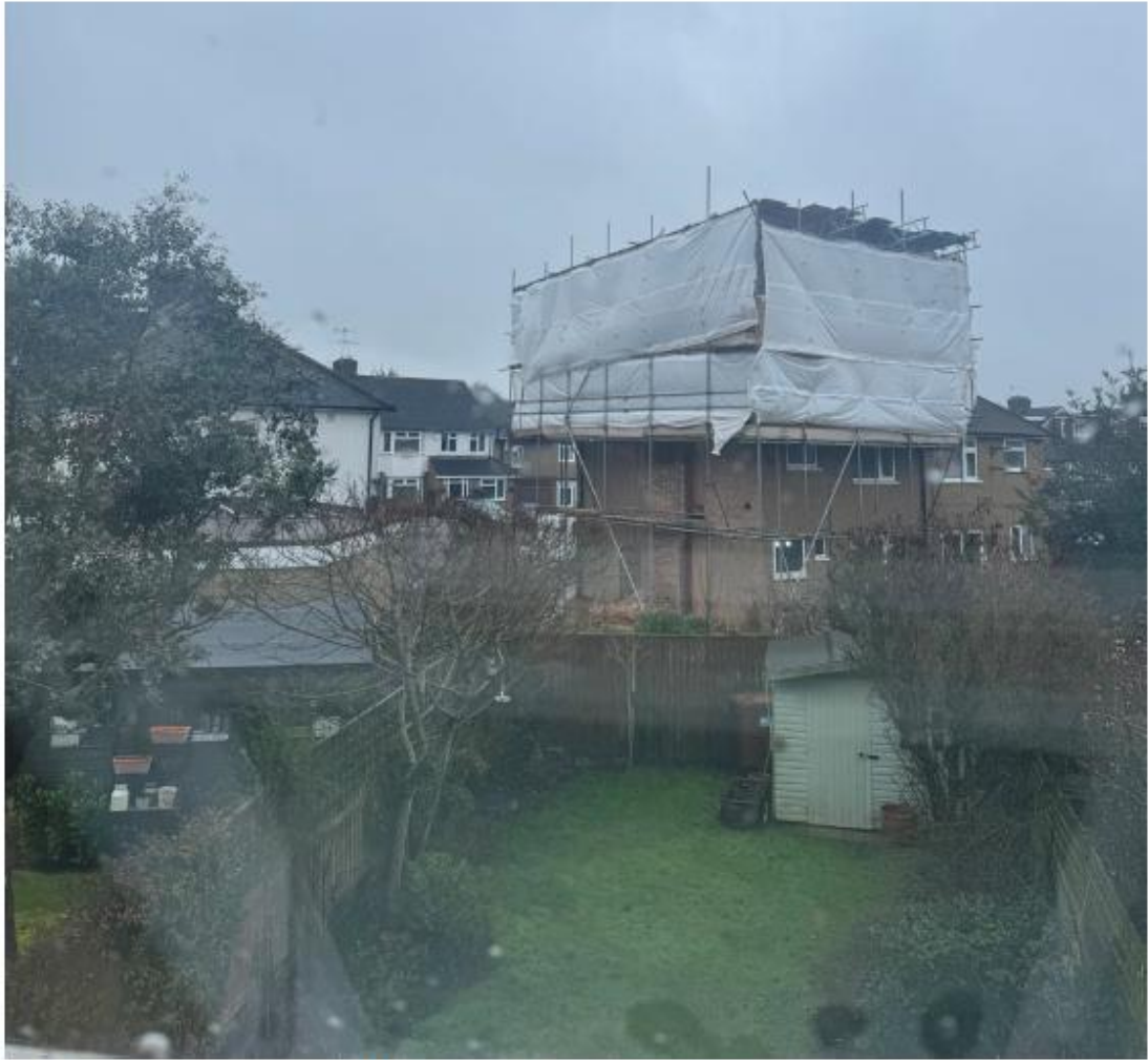
Figure 5: View from 5 Cherry Croft First Floor Rear Window
