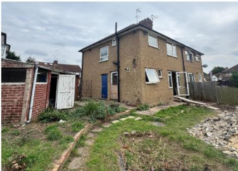
Figure 1: October 2025 Pre Existing Rear Elevation
