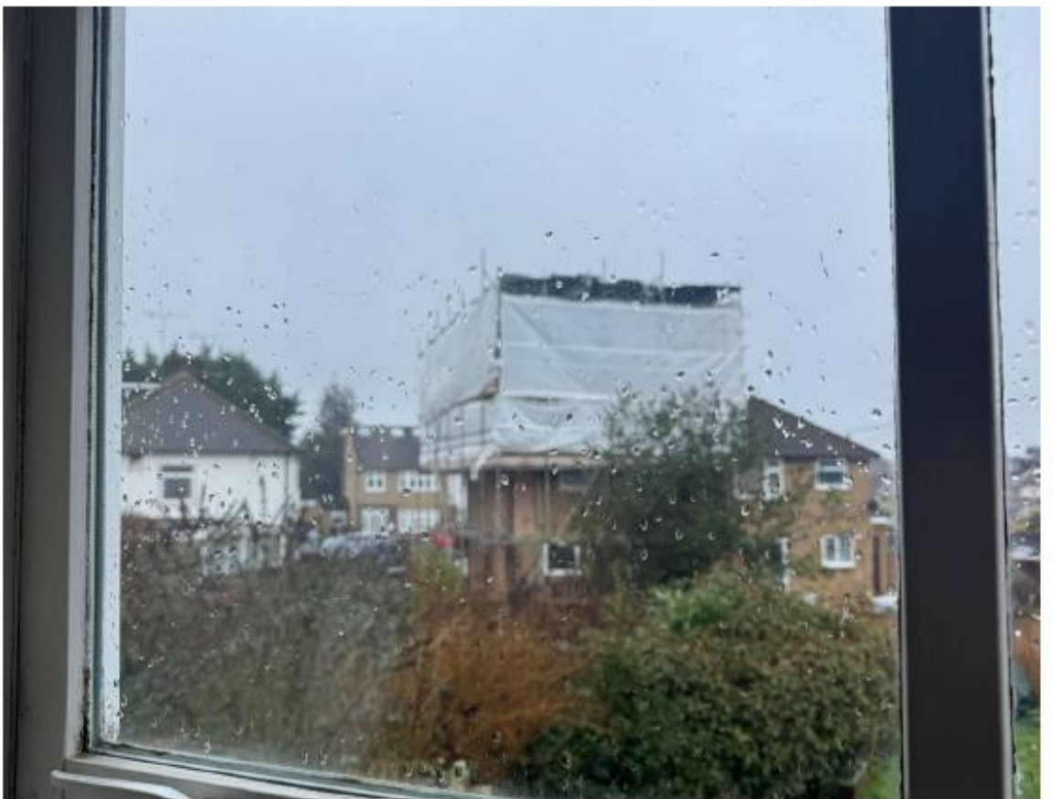
Figure 7: View from 7 Cherry Croft First Floor Rear Window
