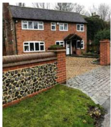
Figure 73: New wall using a mix of traditional local materials © Sarratt Parish Council.
