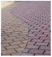
Figure 90: Permeable brick paving.
