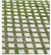
Figure 91: Permeable concrete paving.
