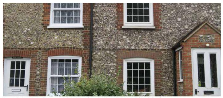
Figure 69: Façades with a consistent arrangement of multi-panewindows with attractive brick ornamentation and articulations.
