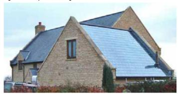
Figure 84: Integrated design for solar panels.
