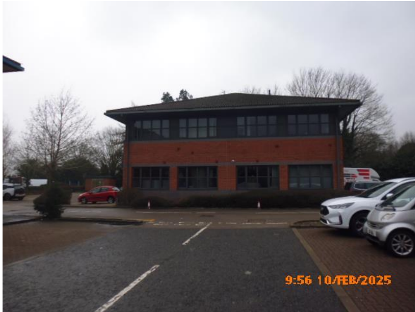
Century House (formally Unit 1)
