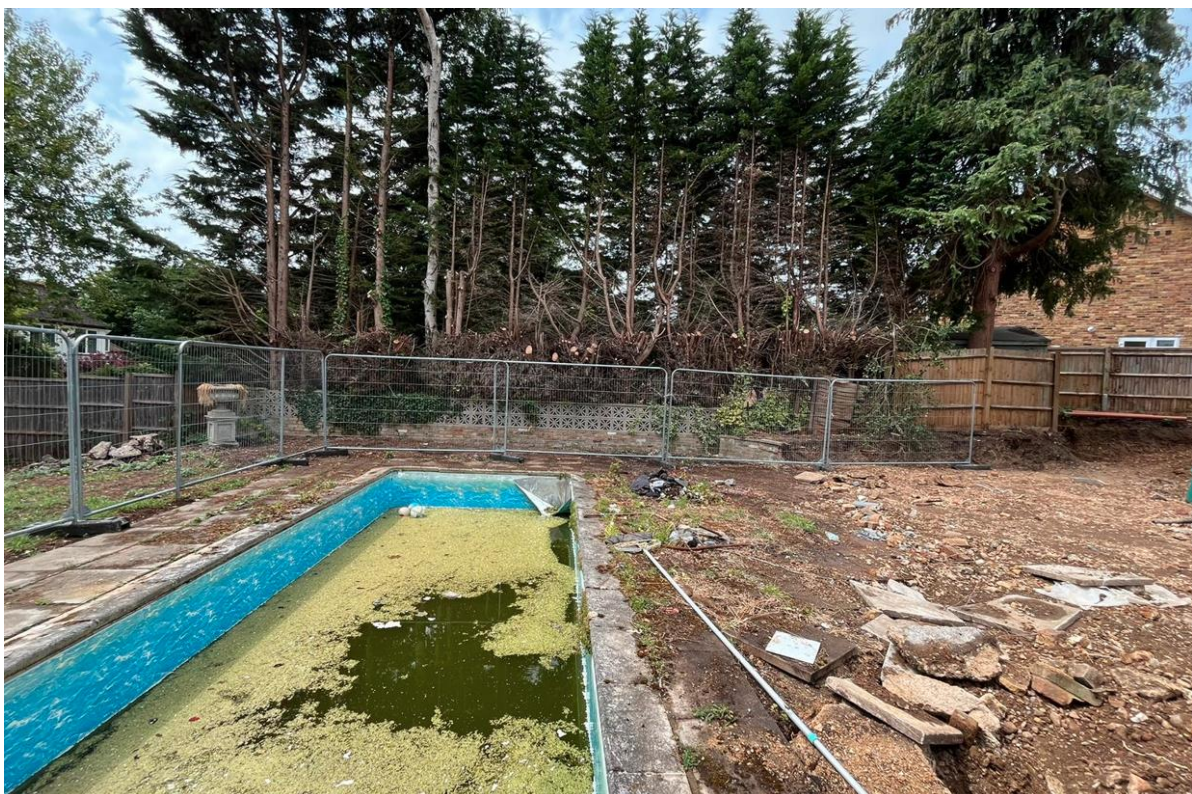
Protective fencing in place on boundary with No. 22 and to rear garden / no equipment on site
