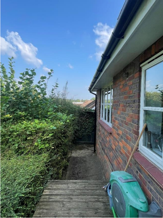
View of 56 Clements Road from existing raised decking.
